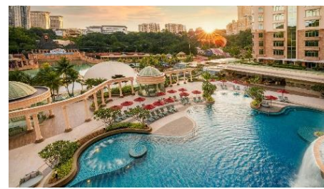
Sunway Resort Hotel Refurbishment
