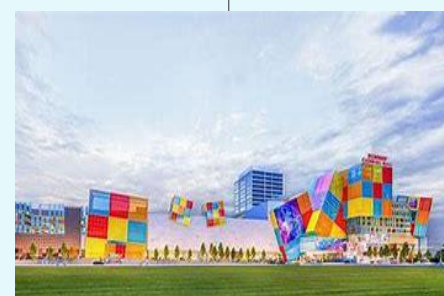
Sunway Carnival Mall Existing Wing
